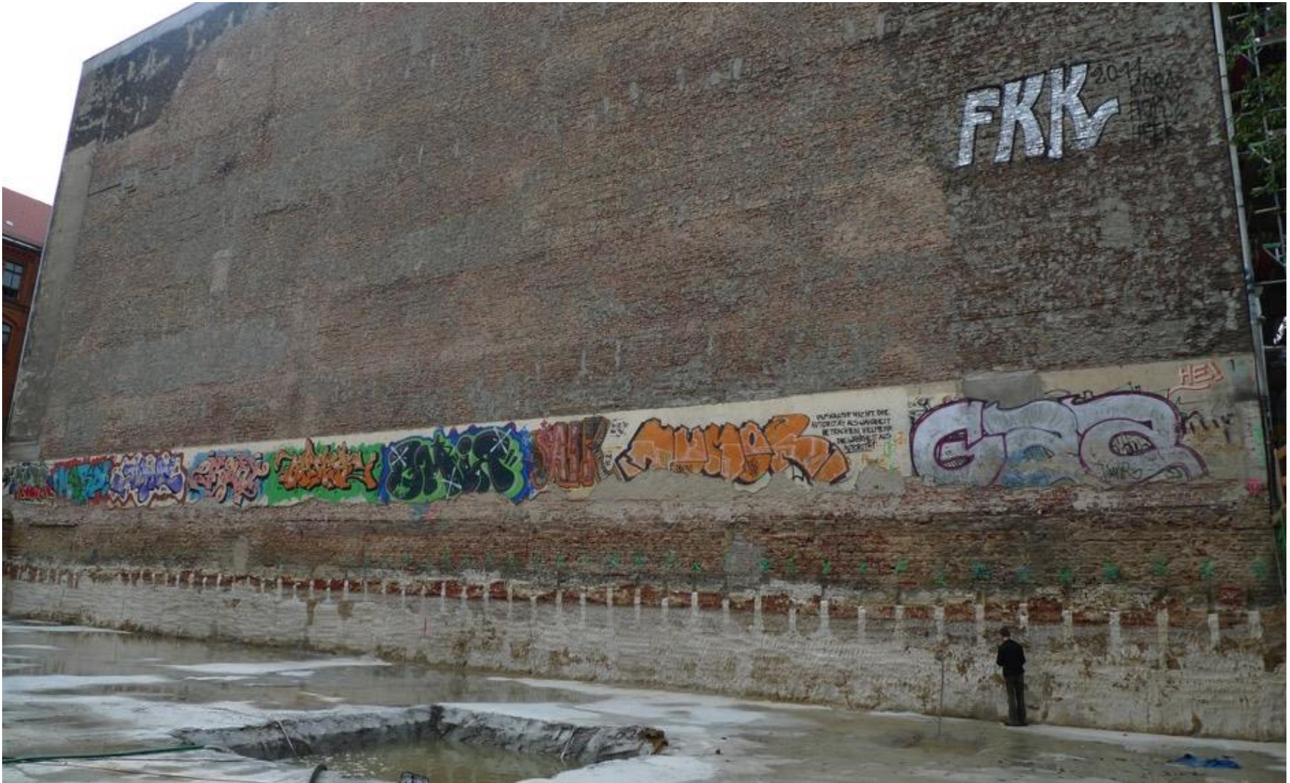
Christburgerstr. 13, Berlin, 2013; Kaden Klingbeil, Architects; Pirmin Jung, Engineers Winter / bauart, check engineers
